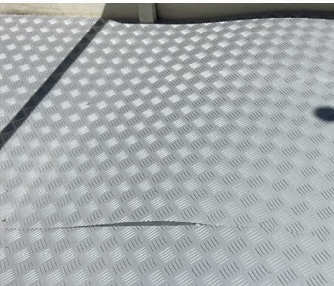
Figure 1: The result of not allowing for thermal expansion is bowing or buckling of the floor
