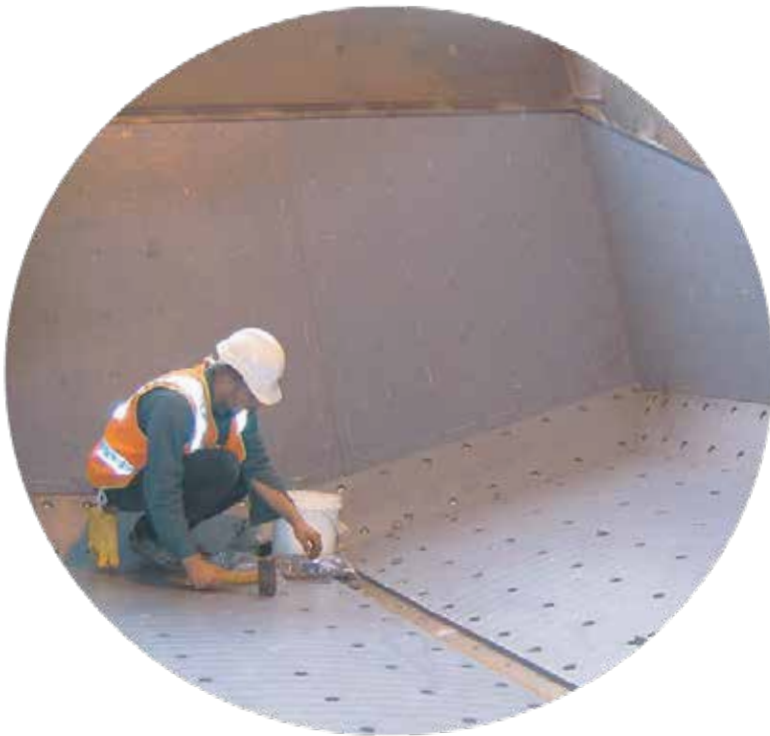
Installation of Matrox Truck Flow Promotion Lining
